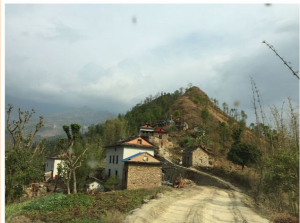
Poku, Ramechhap: the home owner has built a one room, one storey ‘earthquake-safe’ building next to their old, damaged house to access the GoN housing reconstruction grant. They continue to live in the old house because the new one is too small for the family. Photo Credit: Subash Karki/BBC Media Action
