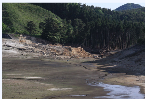
The Fujinuma Dam's empty reservoir.
